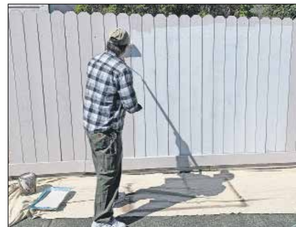
GOOD DEED, INDEED — HSRC facilities supervisor Dave Gaddis paints out graffiti that marred a neighbor's fence. Tasha Romo photo.
